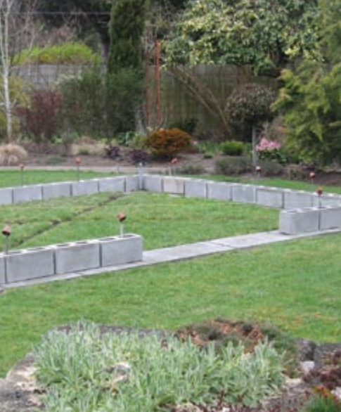
Above, cinderblock and below, brick foundations.
